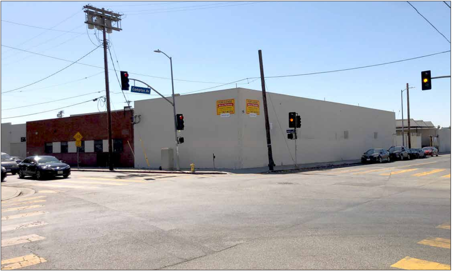
Corner View of Exterior
